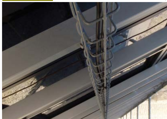
Cable trays - Before specifying and using cable trays to protect and manage conductors within the PV array, check with your local AHJ. Currently, the NEC does not allow cable trays in applications...
