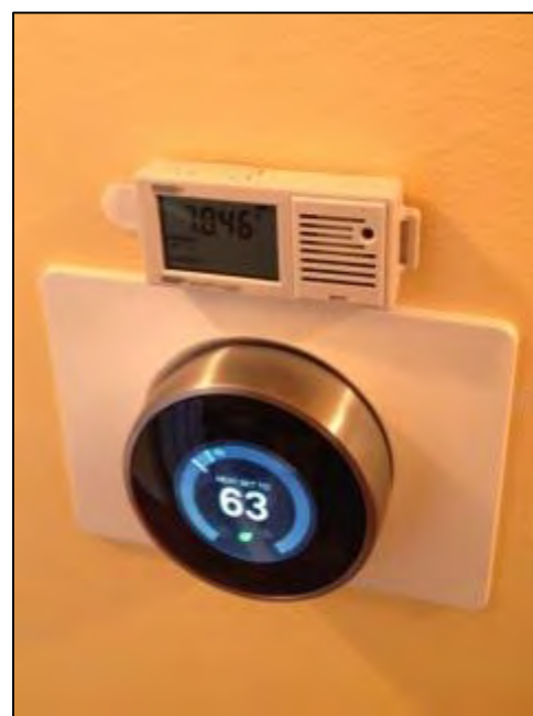
Figure 27. Thermostat Logger Installed Near Programmable (left) and Nest (right) Thermostats
