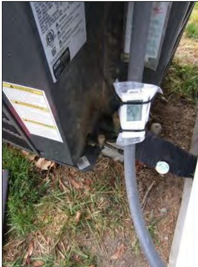
Figure 29. Motor Logger on Electric Conduit to Condenser
