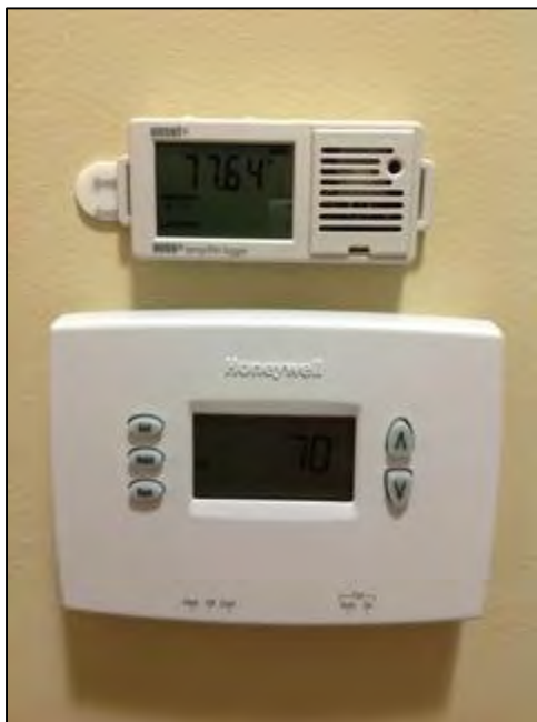
Figure 27. Thermostat Logger Installed Near Programmable (left) and Nest (right) Thermostats
